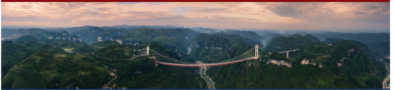
Aizhai Bridge | 矮寨大桥
